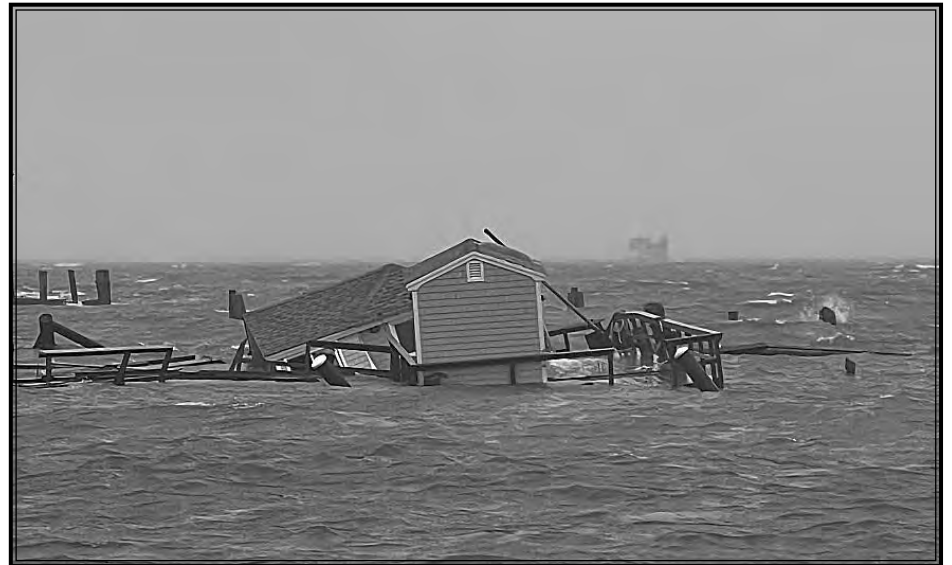
Rebuilding wharves and structures, like this one in Rockland harbor during the January 13 storm, requires hard decisions about what the future might bring. Maine Public photo.
